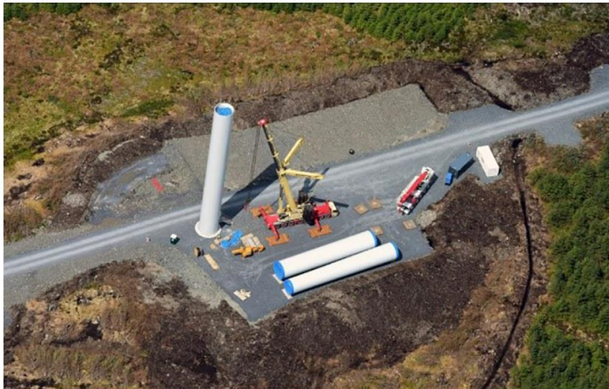
Above: Tower construction at SPR's Kilgallioch Windfarm
