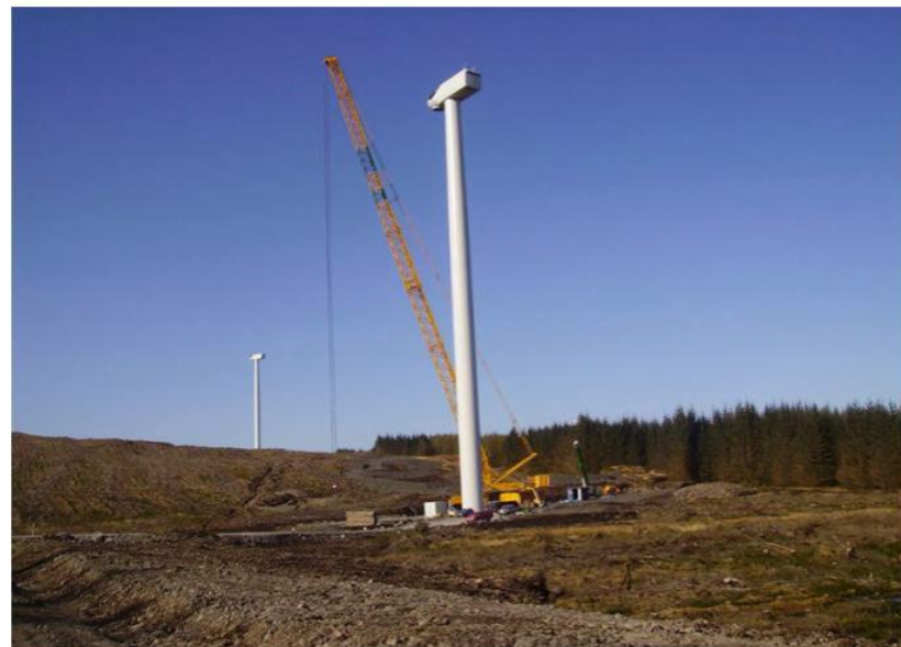
SPR's Kilgallioch Windfarm during construction. Turbines in image are 180 metres tall. The proposed turbine height at Harestanes South will be up to 200 metres to blade tip.
